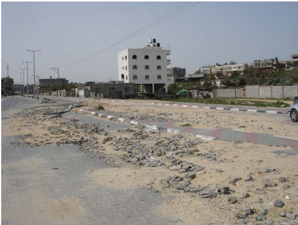
Main Road and street lighting
