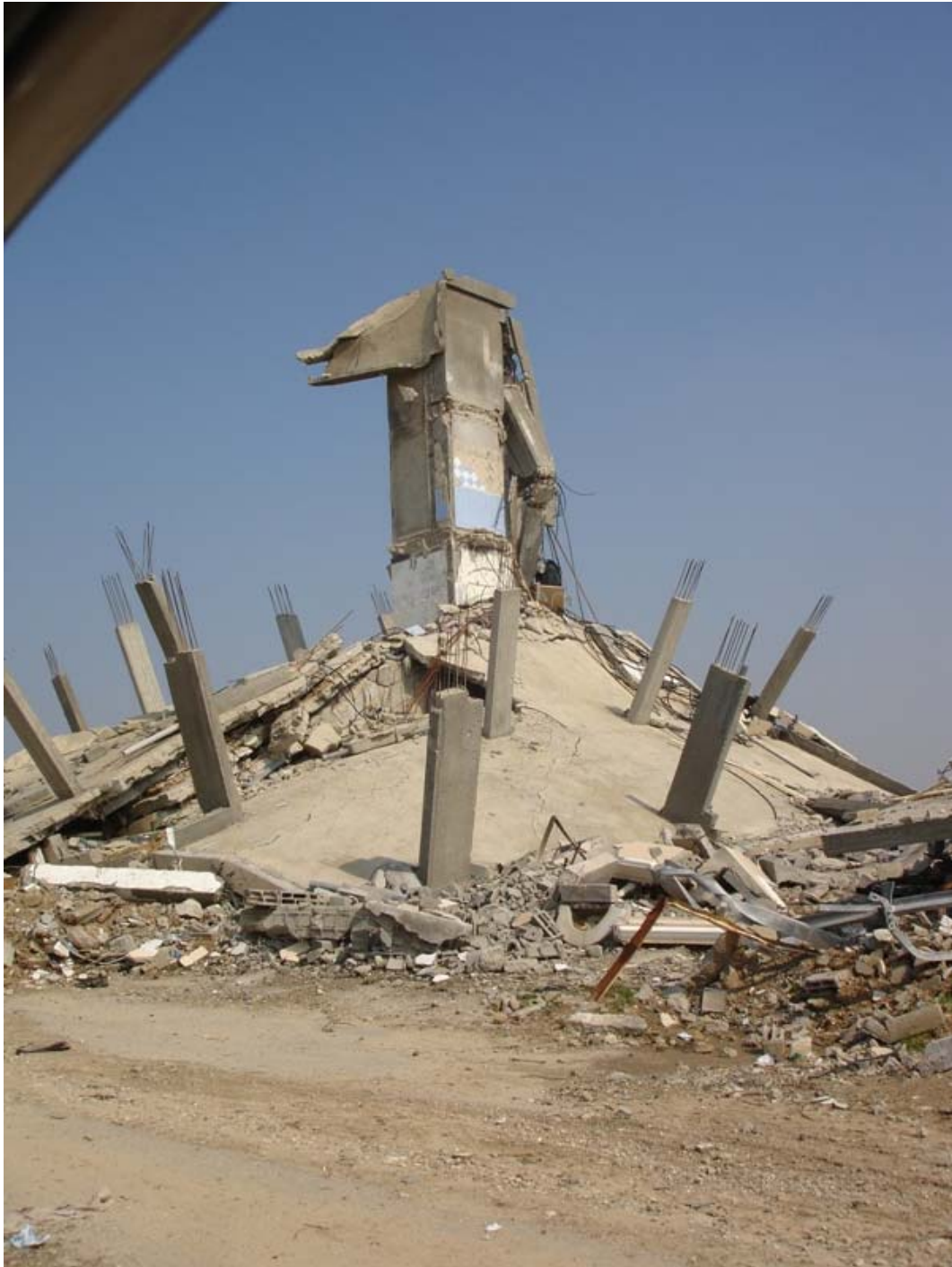
Residential multi storey building
